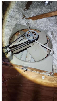
Attic fan appears to be functioning properly.
