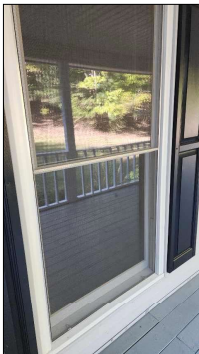
Components appeared in satisfactory condition at time of inspection.
