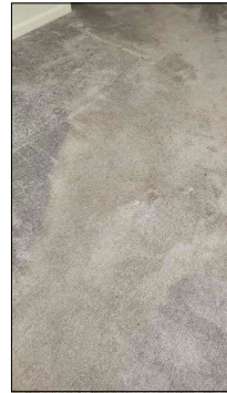
Carpet has stains in various places - recommend cleaning first, if not satisfied, change for new carpet or other flooring.
