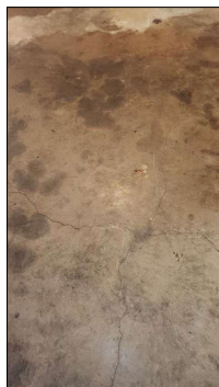
Bare concrete floor in basement.
