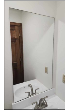
Mirrors were in place and appear to be in good condition.
