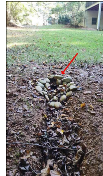
Grade drain termination point noted.
