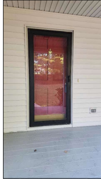
Front door looks to be in good condition and worked properly during inspection.
