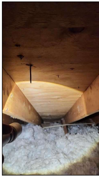
Under eave soffit inlet vents noted.
