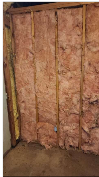
Insulation in place.
