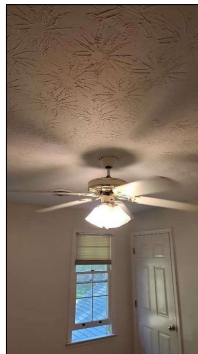
The ceiling fan in one guest bedroom is a worn unit that has reached the end of its useful life.
