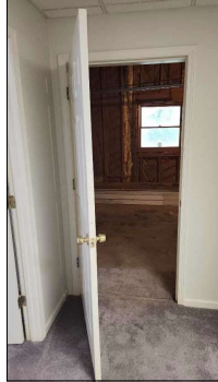
Internal entry is in good condition.
