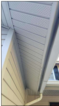
Eaves and facia in good condition at time of inspection.
