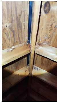
Ridge exhaust venting noted.
