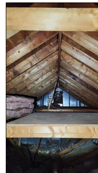
Attic rafters and sheathing appear to be in good condition.
