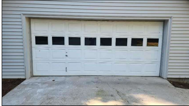
Garage door looks good and functioned properly.
