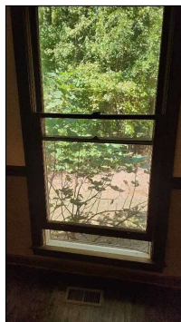
Windows worked properly during inspection.
