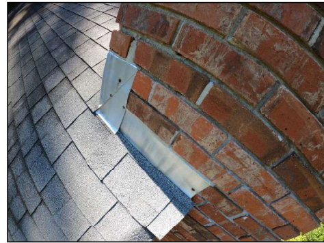
Flashing in place and appears functional.
