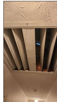
Attic fan appears to be functioning properly.
