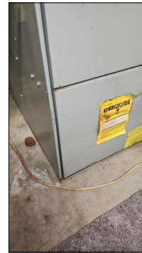
None at basement noted.
