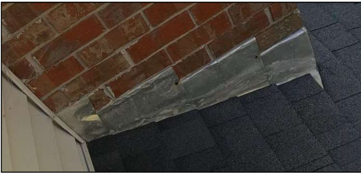
Flashing in place and appears functional.
