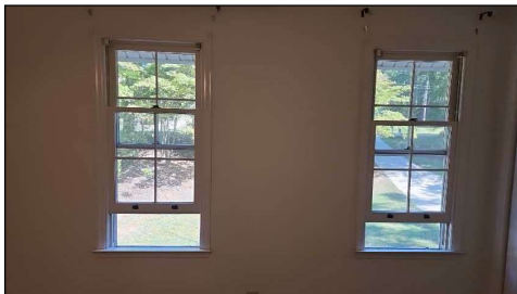
Windows operated properly when tested during inspection.
