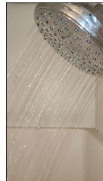
Worked properly during inspection.
