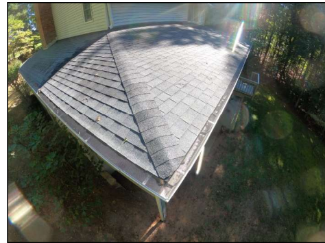
No major system safety or function concerns noted at time of inspection.
