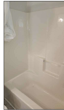
Fiberglass surround noted.
