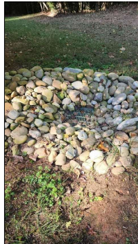
Grade drain noted.
