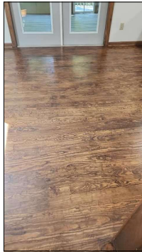
Hardwood floor looks to be in good condition.
