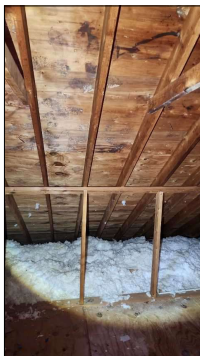
Attic rafters and sheathing appear to be in good condition.
