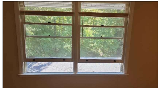
Windows operated properly when tested during inspection.
