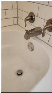
Tub functioned properly during inspection - no drain issue noted.
