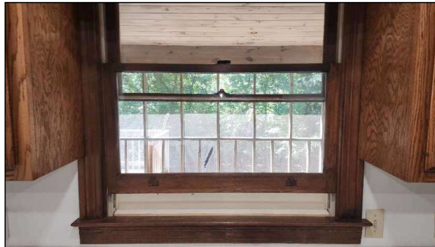
Windows functioned properly.
