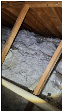
Insulation appears adequate.
