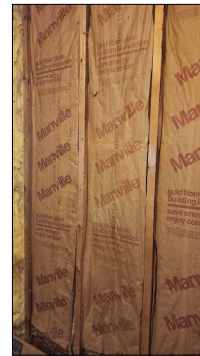
Insulation in place.
