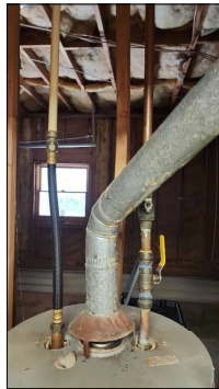
No major deficiencies observed at the visible portions of the supply piping.
