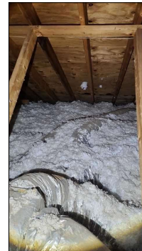
Insulation appears adequate.
