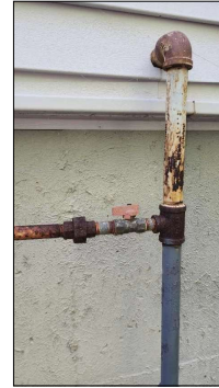
Rusting noted at pipes.
