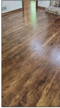
Hardwood floor looks to be in good condition.
