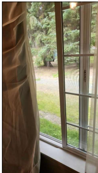
Windows operated properly when tested during inspection.
