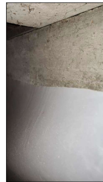
Foundation walls look good.
