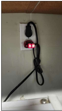
Outlet functioning properly.
