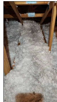
Insulation appears adequate.
