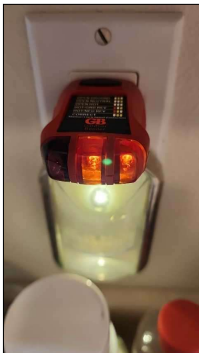
GFCI in place and operational
