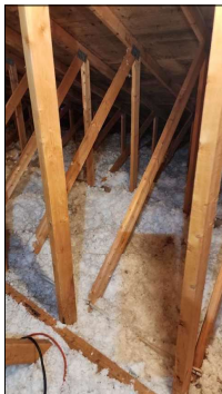
Insulation appears adequate.
