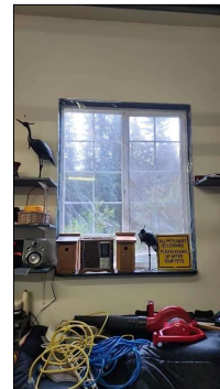
Windows were functional.
