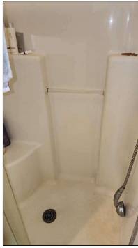
Fiberglass surround noted.
