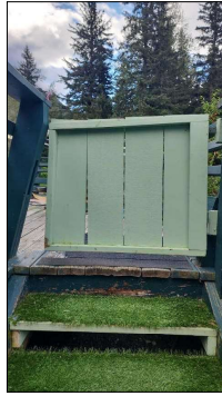
Gate was functional.
