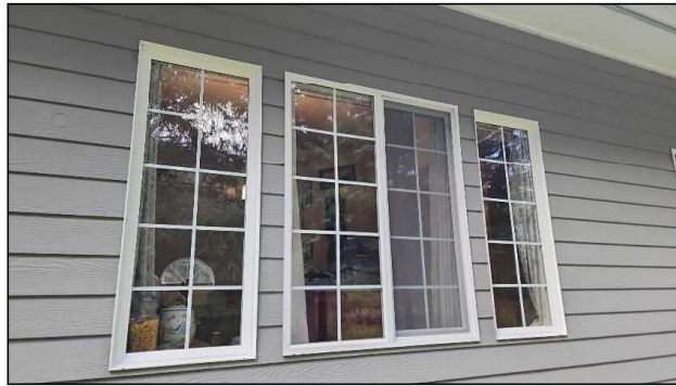
Components appeared in fair condition at time of inspection.
