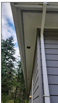
Eaves and fascia in good/fair condition at time of inspection.
