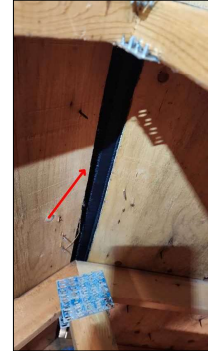
Ridge exhaust venting noted.
