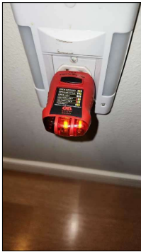
Outlet functioning properly.
