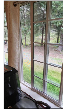
Windows worked properly during inspection.
