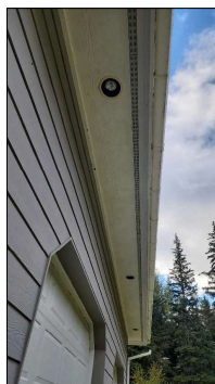
Eaves and fascia in good/fair condition at time of inspection.
