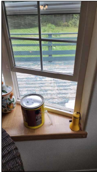
Windows worked properly during inspection.
