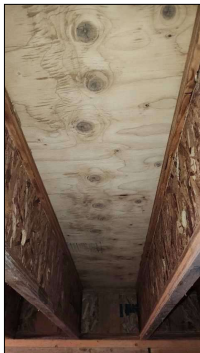
Visible parts of subfloor appear to be in good condition.
