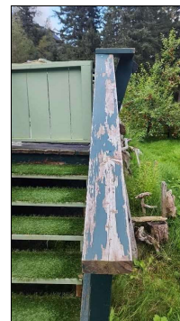
Recommend paint or stain to preserve.
