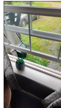
Windows operated properly when tested during inspection.
