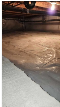
Plastic vapor barrier noted.
