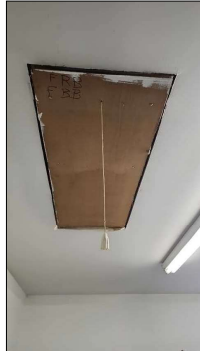
Pull Down Ladder located in: Garage
