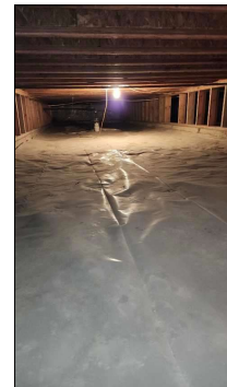
Plastic vapor barrier noted.
