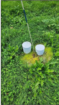
Septic system noted. Client is advised to seek the services of a specialist in evaluating this system.
