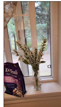
Windows worked correctly when tested during inspection.
