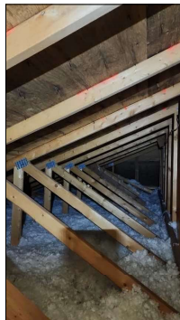
Attic rafters and sheathing appear to be in fair condition.
