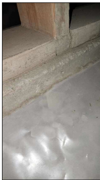
Foundation walls look good.
