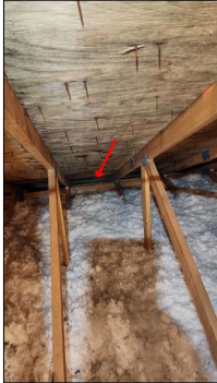
Under eave soffit inlet vents noted.
