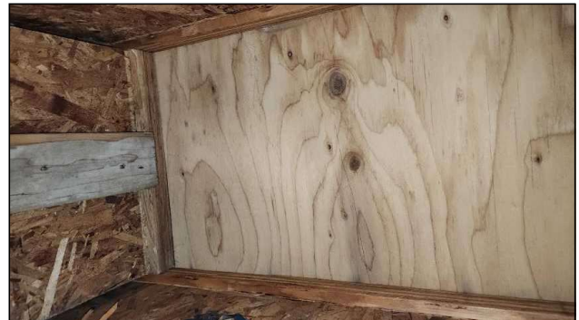
Visible parts of subfloor appear to be in good condition.
