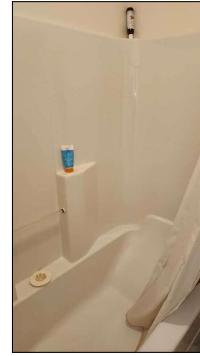
Fiberglass surround noted.
