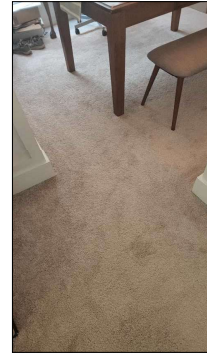
Carpet in fair condition.
