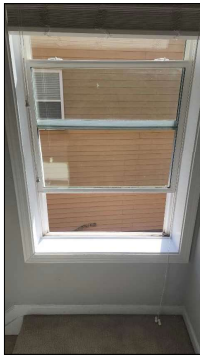
Windows worked properly during inspection.
