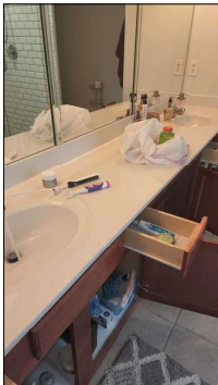
Composite tops noted.
