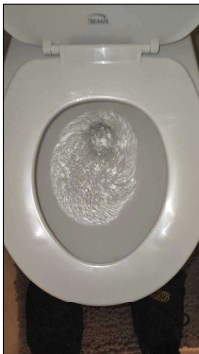
Observed as functional and in good visual condition.
