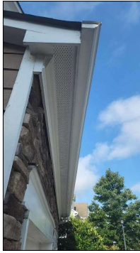
Eaves and fascia in fair condition at time of inspection.
