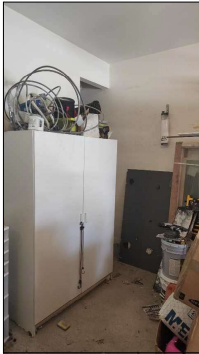
Visible walls look fair.
