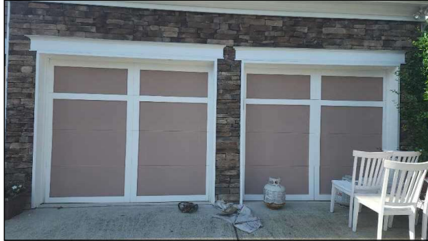
Garage door looks good and functioned properly.
