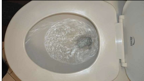
Observed as functional and in good visual condition.
