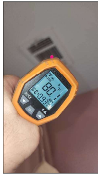
Heat did not function properly when tested at second floor. Recommend evaluation and corrections by a licensed HVAC specialist.
