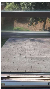
Windows operated properly when tested during inspection.
