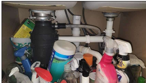
Plumbing looks to be in good condition. No apparent issues noted.
