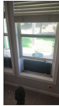
Windows worked properly during inspection.
