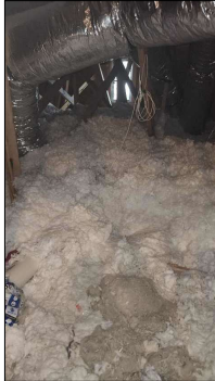
Insulation appears adequate.
