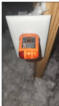
Outlets functioned properly during inspection.
