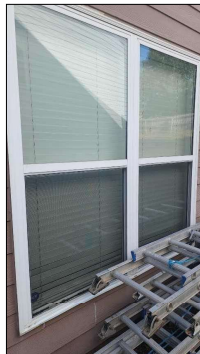
Components appeared in satisfactory condition at time of inspection.
