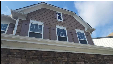
Components appeared in satisfactory condition at time of inspection.
