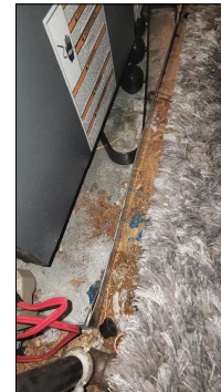
The heater base appears to be functional.
