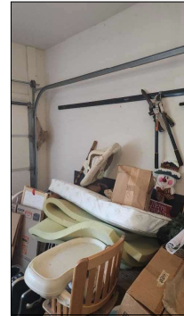
Visible walls look fair.
