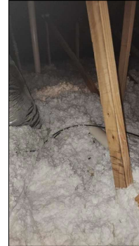
Insulation appears adequate.
