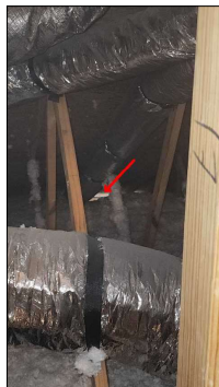
Under eave soffit inlet vents noted.
