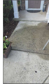
Walkway was in fair condition.
