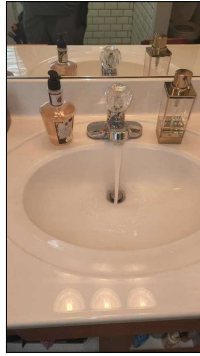
Operated normally, at time of inspection.
