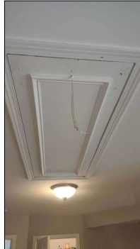
Pull Down Ladder located in: hallway
