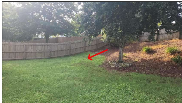
Backyard slopes toward the house.
